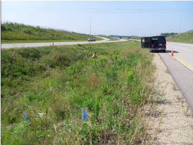
Fig. 1. The Roadside drainage ditch on Hwy 212 near Chaska, has been shown to infiltrate stormwater and act as a grassed swale.
